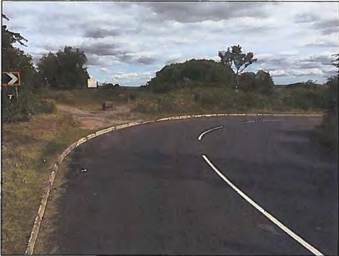
Photograph showing Chevron plate that has slipped down posts - looking west
