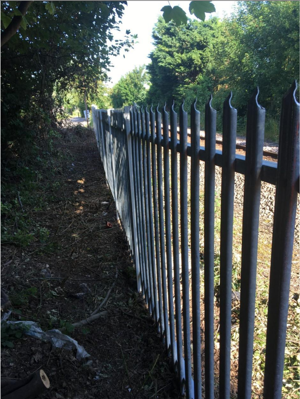
PHOTO 4 – New Upside Fencing looking back towards Fulburn Old Drift Rd.
