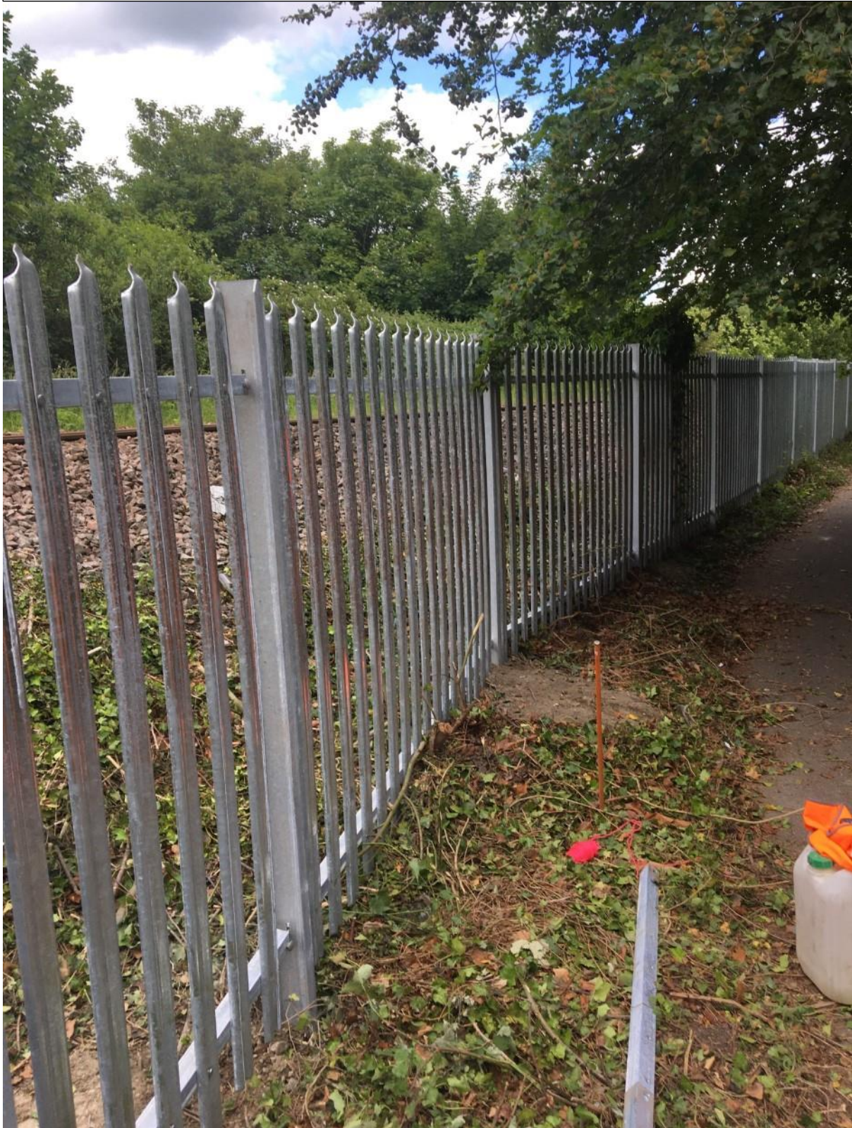
PHOTO 3 – New Upside Fencing linking up with existing fencing at the Fulburn Old Drift Rd
