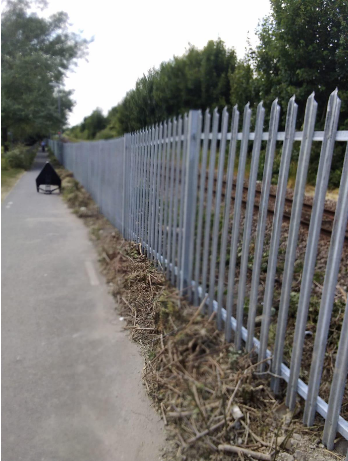
PHOTO 1 – New upside fencing looking towards Cherry Hinton
