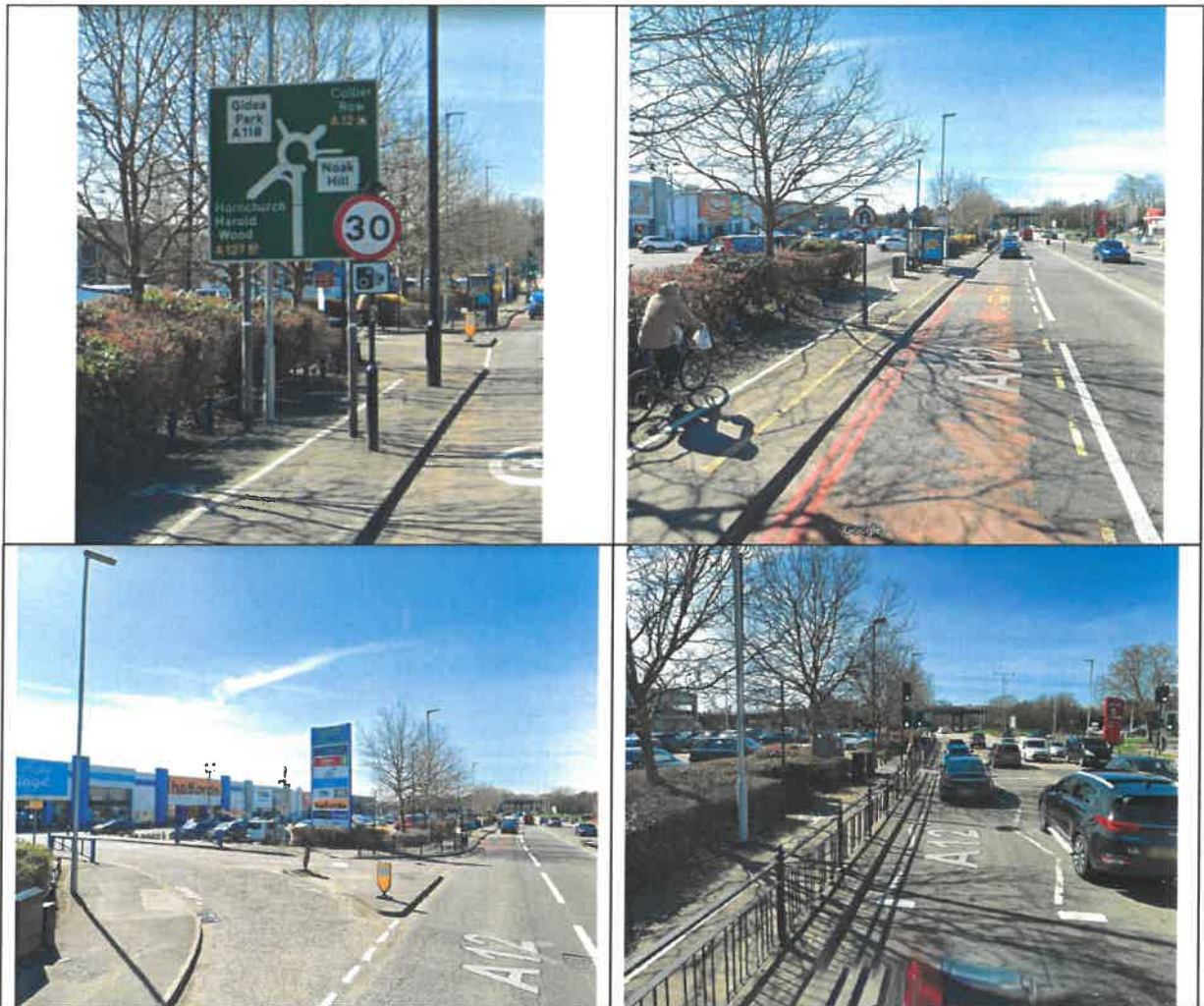
Signage in the vicinity of the controlled crossing point
